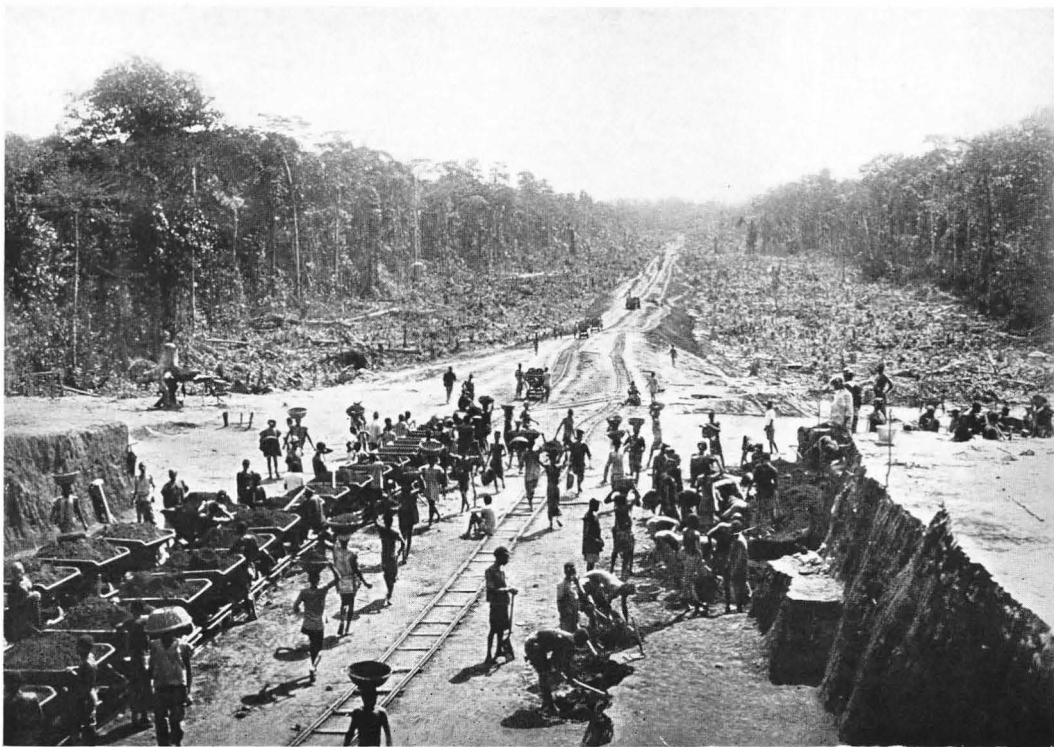
RAILWAY CONSTRUCTION THROUGH THE IMO SWAMP
